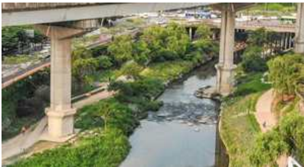
< Before Bridge Construction >
