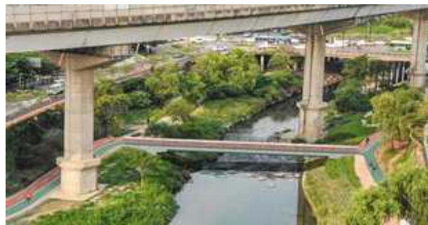
< After Bridge Construction >
