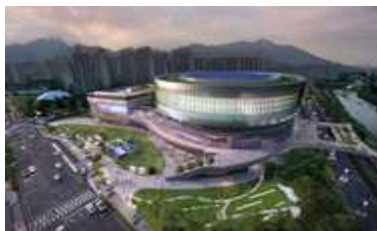
Seoul Arena (scheduled to open in 2027)
